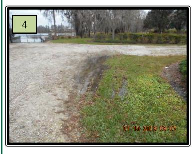
**4. Reference Pic (4)** Located to the left hand side of amenities center along boat ramp driveway there is a main line break that needs to be repaired. Main line breaks need to be repaired as soon as possible so irrigation is not down long.
